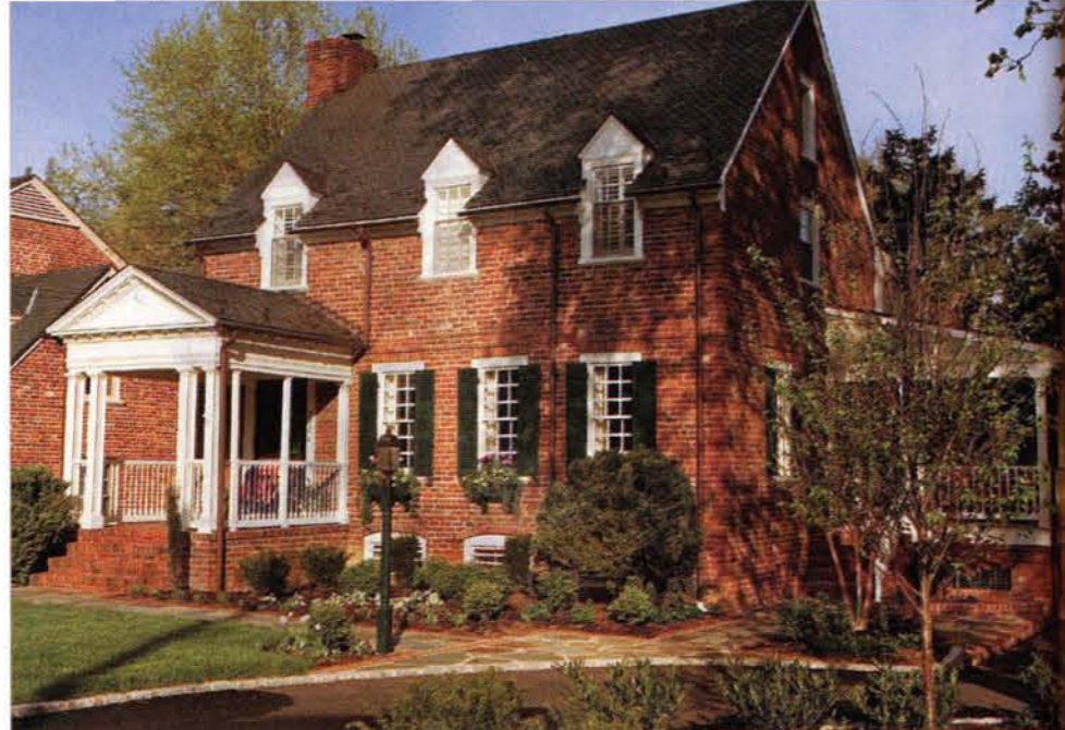
TOP RIGHT: The original walkway cut through the middle of the front yard. Landscape designer Robin Woods rerouted the walkway, which now connects the new driveway along the side of the house with the front door.
